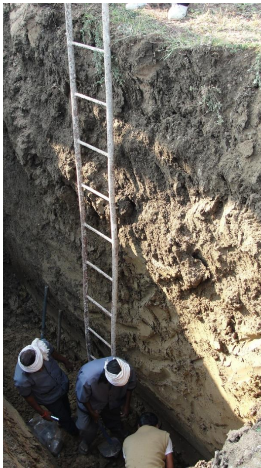
Fig. 12 Geotechnical Investigations in IIIT, Basar
