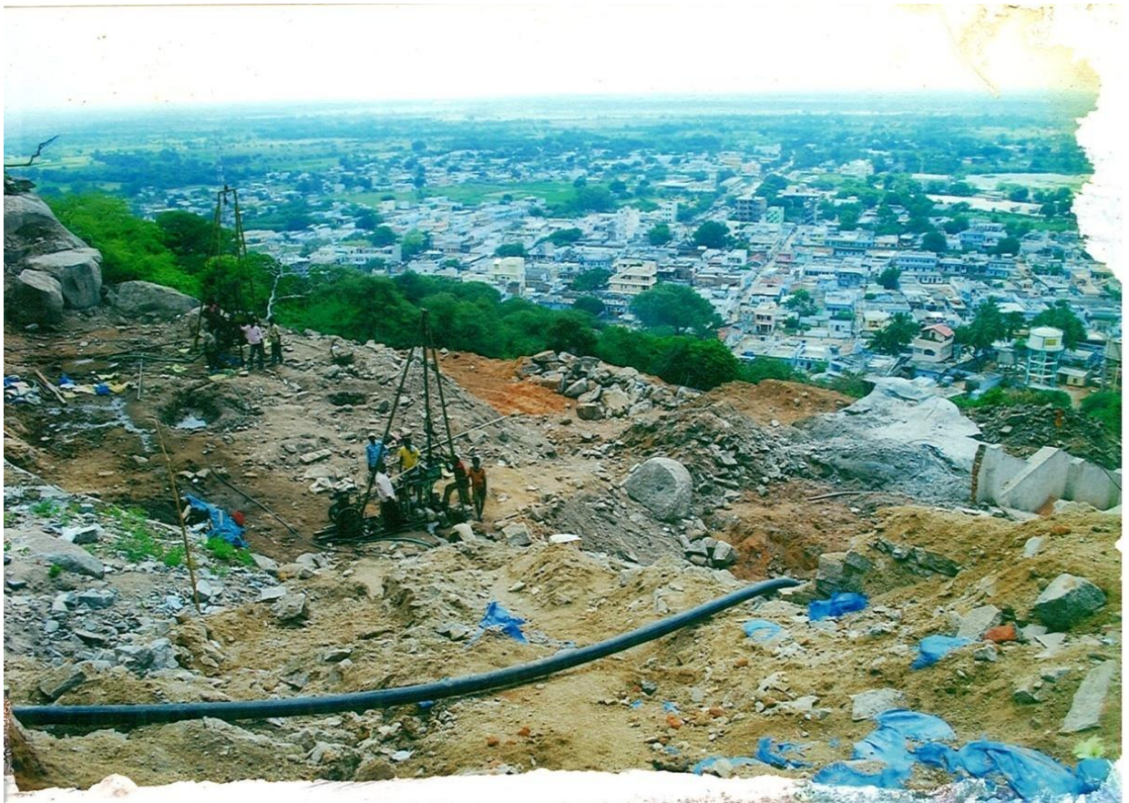
Fig. 10 Geotechnical Investigations in Yadagirigutta Temple Shrine in progress
