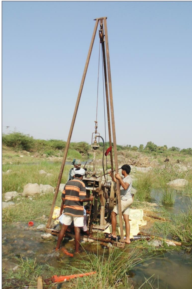
Fig. 13 eotechnical Investigations for construction of a Bridge near Peddavura (v)
