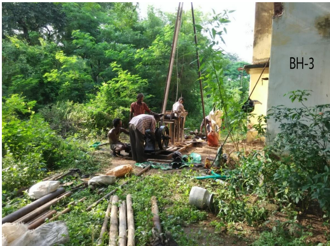
Fig. 14 Geotechnical Investigations for Super Specialty Block in KIMS, WARANGAL
