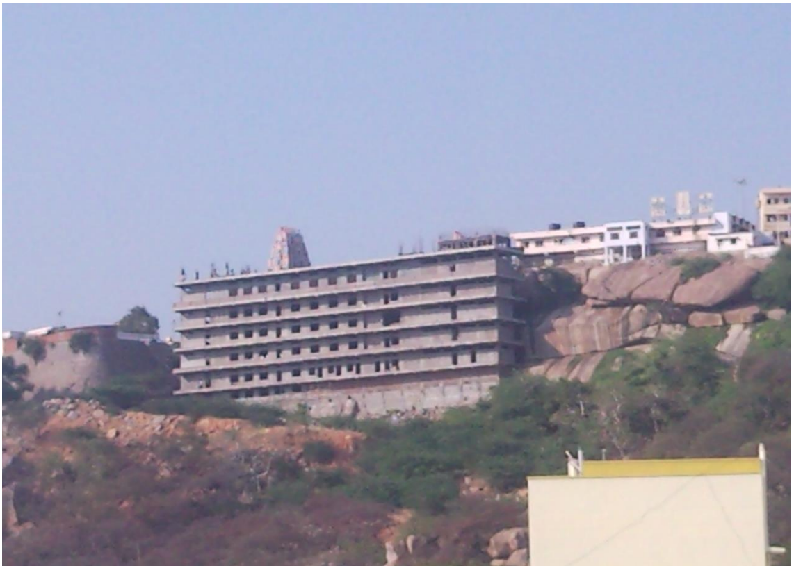
Fig. 11 Construction of South Side Block in Yadagirigutta Temple shrine
